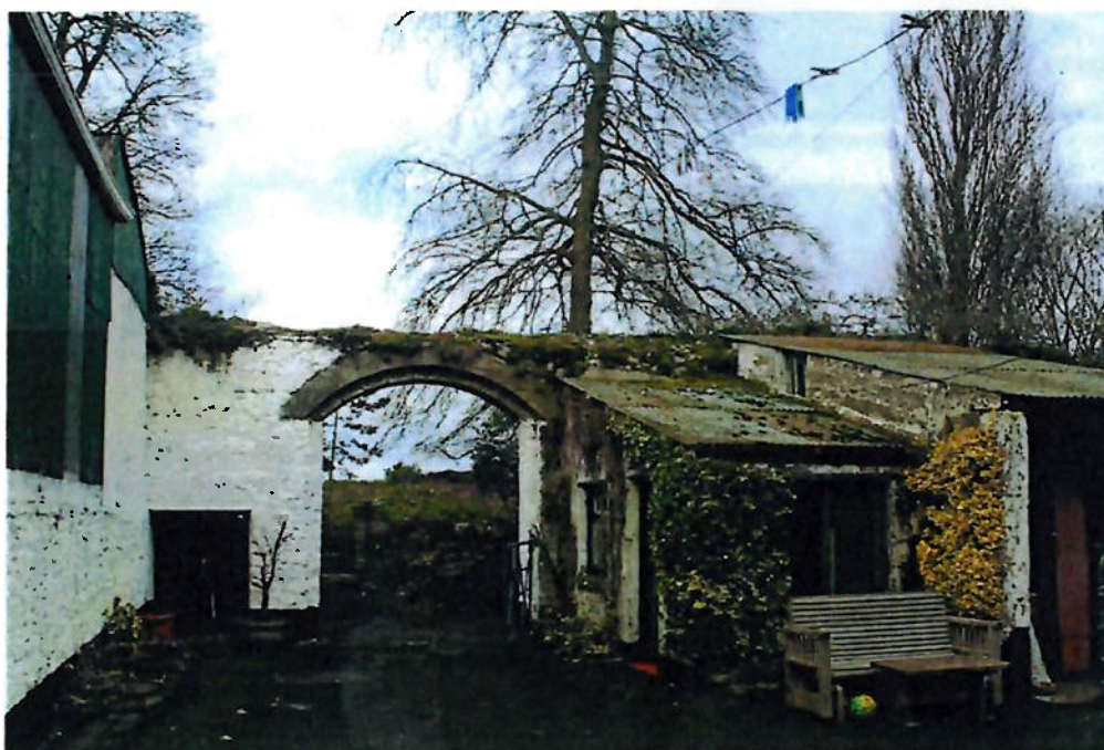
fig 18 Entrance arch to rear yard.
