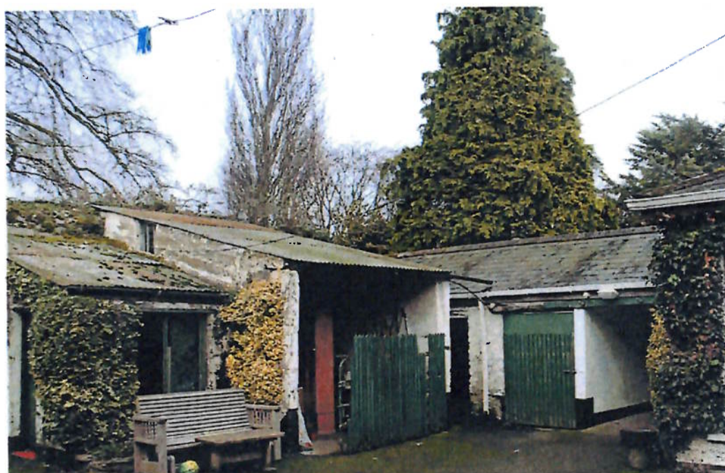
fig 20 Outbuildings to north of house
