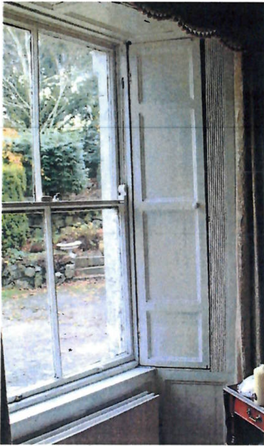
fig 15 Shutters in south bow showing fluted detail.
